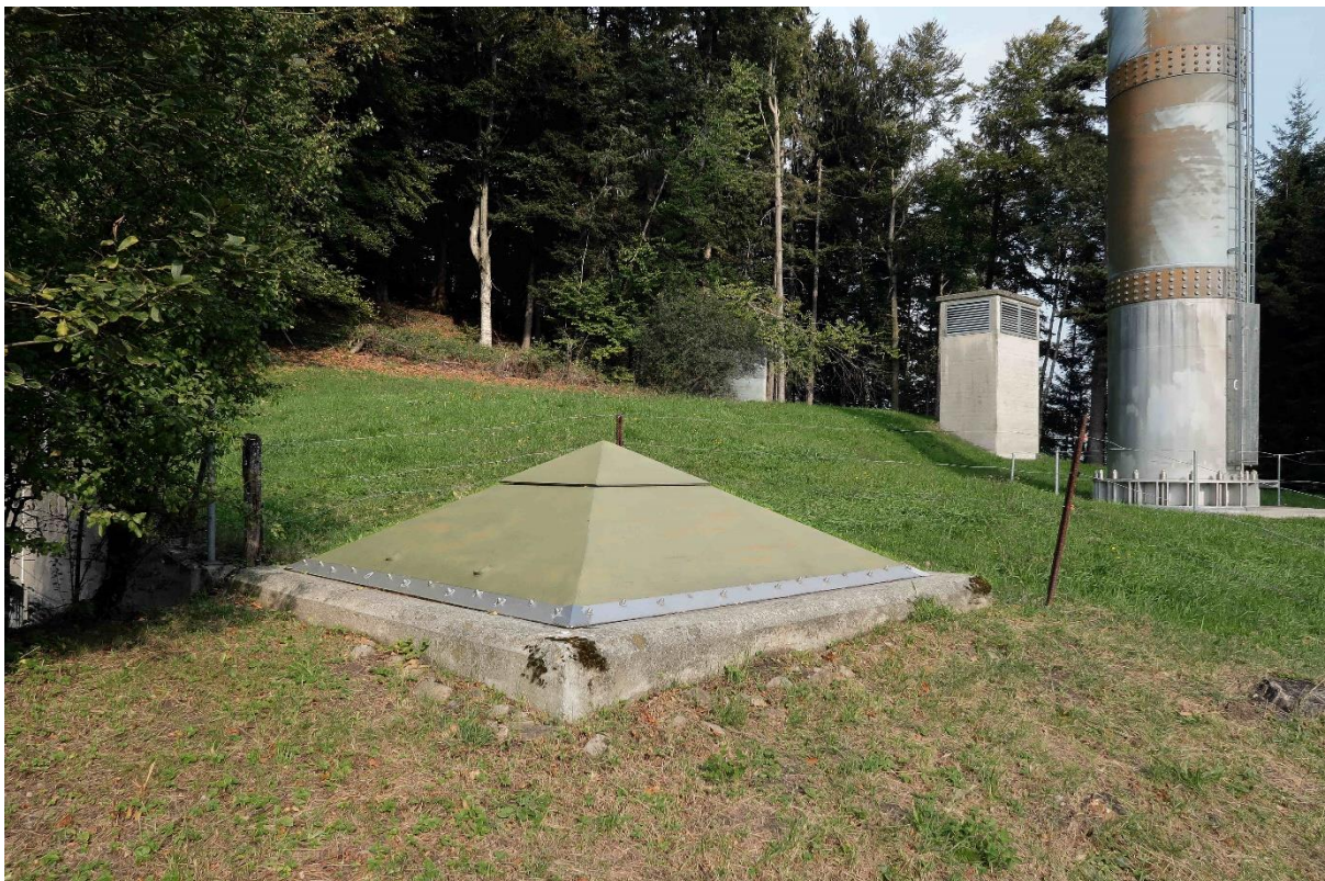
IBBK-Sendeanlage: rechts Betriebs-Antenne, links Not-Antenne. Von Kecko from Rural area of Eastern Switzerland - IBBK-Radio Pyramid, CC BY 2.0, https://commons.wikimedia.org/w/index.php?curid=73382401
